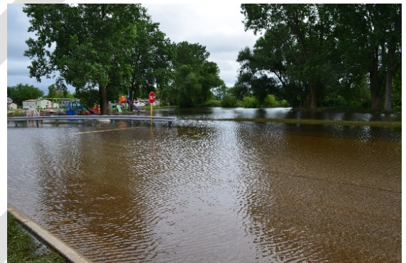
Figure 2-3: City of Park City July 2017 roadway flooding along the Dady Slough
