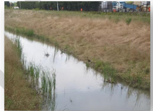
Figure 2-3: Skokie River Stream Daylighting Project, Two-Stage Channel
