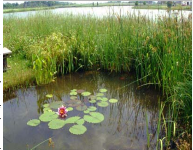
A typical stormwater wetland at the edge of a wet basin.
